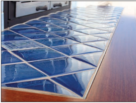
1.1 Schluter®-SCHIENE , in satin anodized aluminum, installed to protect tile edges and provide a clean transition to surrounding hardwood flooring at the same elevation.
